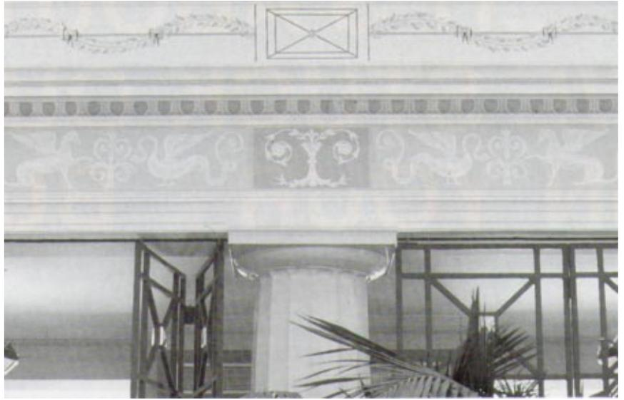
*Veneer plaster was used to recreate an array of intricate details in the Stouffer hotel's original plaster work and columns.*
